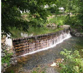
1790 timber crib dam, Green River, Vermont
